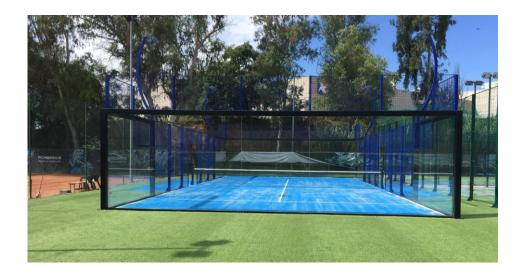
The side elevations will incorporate a central opening for player access on one or both sides, or where the out of court play area (8.00m x 2.00m overall) is to be incorporated for elite tournaments. Openings for access may be single or double arrangement. To allow wheelchair access to either end of the court, the spacing between the net post and the enclosure must be a minimum of 1.2m on either side of the court.
